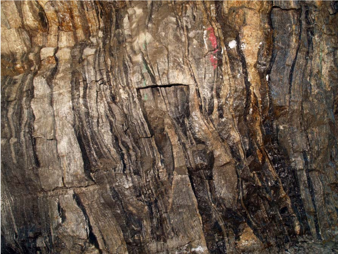
Figure 6 - Typical well-layered and foliated Fordham Gneiss (Yf). Station 5+85, north wall raw water tunnel, Croton Water Treatment Plant, Bronx, New York. (Digital image by C. Merguerian).
