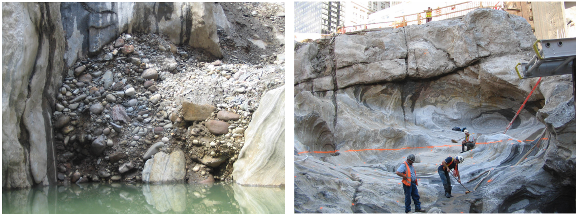
Figure 10 – The bedrock at the World Trade Center site was scoured into deep plunge pools and potholes, especially around the contact zone between schistose rock and large masses of hard granite pegmatite. The plunge pools were then filled with a dense boulder and cobbly till. On the left, the till is still filling the west side of the western plunge pool. On the right, the till has been removed from the east side of the same plunge pool for construction. It is likely that at least the lowest tier of the Manhattanville valley resembles this combination of scoured rock filled with till. (From Moss & Merguerian 2009)
