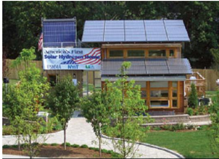
USMMA Solar Hydrogen House King's Point, NY
